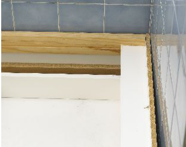
1. PROBLEM: An out of square corner.
