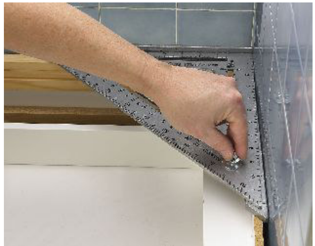
4. Keeping the square in position, tighten the front-most wing nut.
