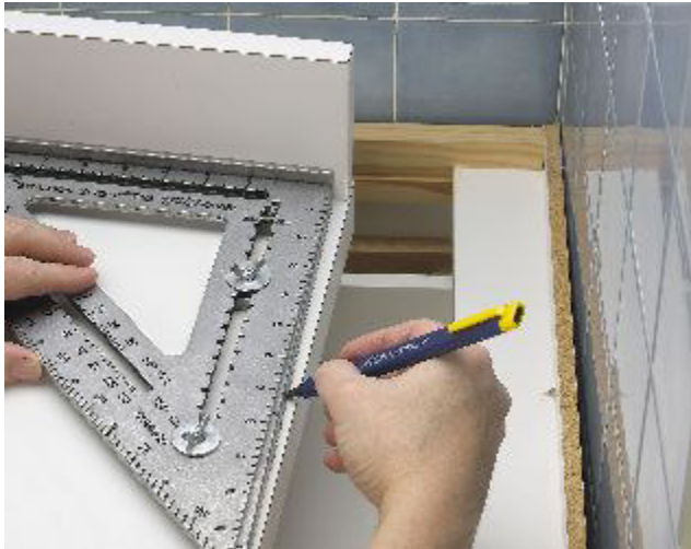
5. Place the now adjusted square on the edge of the countertop and transfer the corrected angle.
