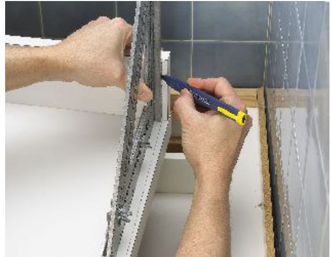
6. Stand the Big 12® Speed® Square to mark the back splash.
